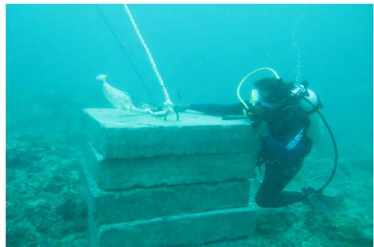
Figure 10. Concrete Ballast deployment for the mooring's anchors
