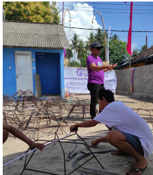
Figure 16. Fish dome and reef star structure for the coral rehabilitation program
