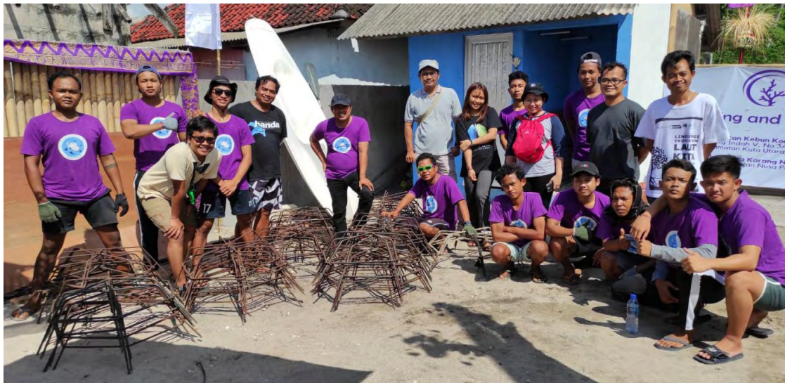
Figure 17. CTC team in the making of the reef structures in Ped Village
