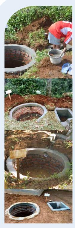
Water catchment wells constructed in the recharge area of Bismo spring with dimensions of 1 meter diameter and 3 meters depth.
