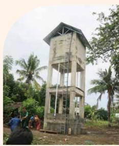
The main water tank that could accommodate water up to 12 m³ is installed in sub-village Tampes Kayangan Village.
